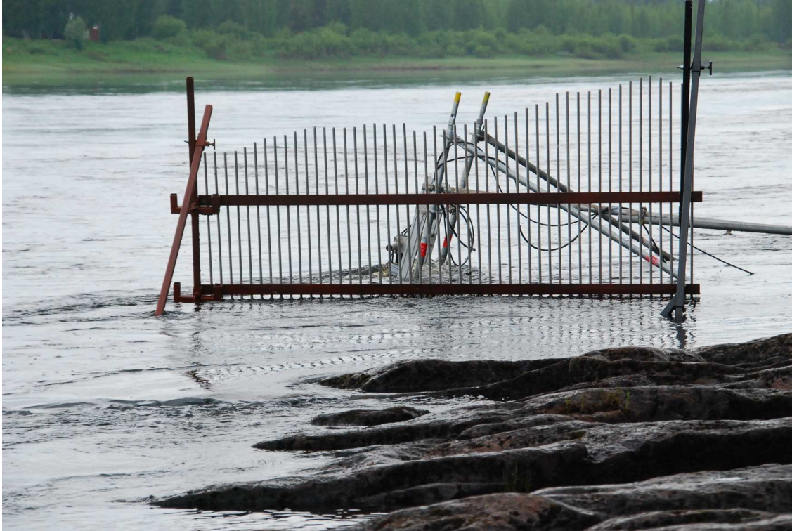
Figure 6. A steel stand for DIDSON and a fish deflection weir in Kattilakoski, Finnish shore.
